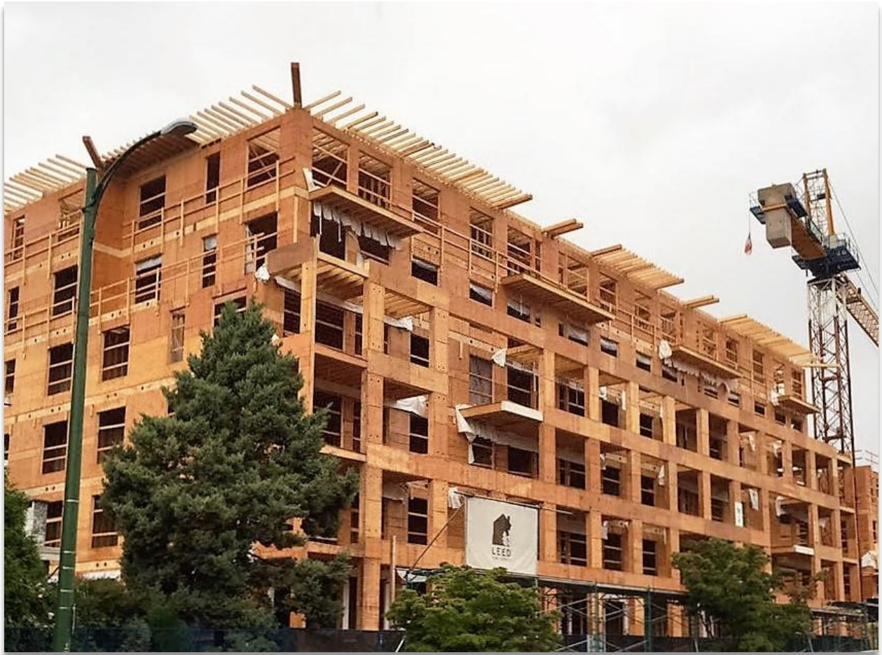
Mid-Rise Wood Frame Building under construction in British Columbia
