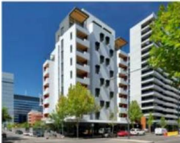
9 storeys - Melbourne Australia, Land Lease
