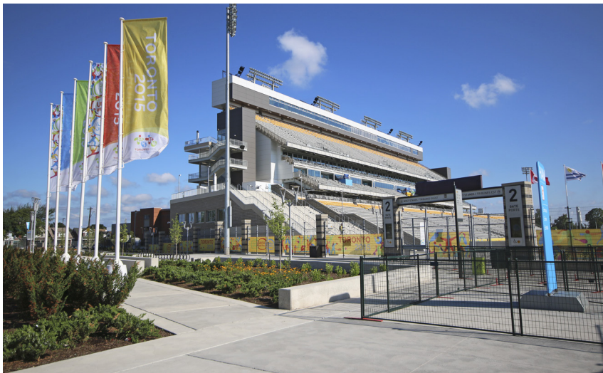
The LEED Silver certified Pan Am Soccer Stadium in Hamilton, ON used lower carbon, Portland limestone cement.
