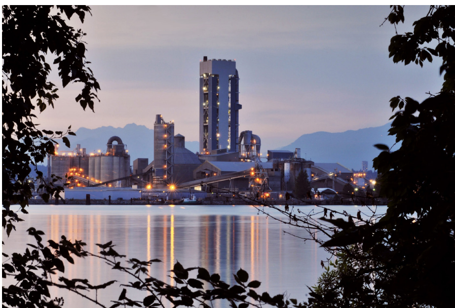
In Richmond, BC Lafarge Canada's CO2MENT carbon capture utilisation and storage demonstrations project has accumulated more than 1000 hours with 85% CO 2 recovery.
